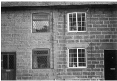
Two cottages at Cromford built by Arkwright for his millworkers c 1780: the left-hand one was given bogus leaded lights in wooden frames c 1989; listed 1990 (DCC)
