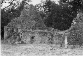
Derwentcote steel furnace before consolidation, viewed from the south: the buttressed furnace with the cone is in the centre; smaller ancillary buildings lie on either side (B Knight)
