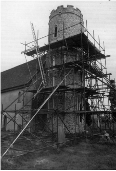
The shoring scaffold and the tower under repair
