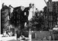
Rear elevation of Manchester Street, following second collapse, May 1990 (Westminster City Council)
