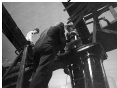
Work being carried out at Fournier Street under exemption
