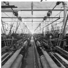
The looms with their overhead drive belts
