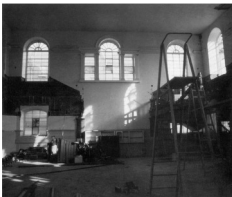
Fournier Street, East London: the gutted interior, 1986
