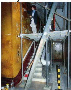
The back staircase during conservation
