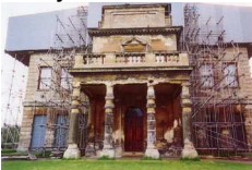
Brodsworth Hall during structural renovations, May 1991
