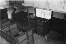
View of the original box pews and the gallery above, July 1992
