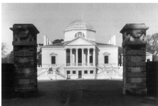
Chiswick House, London, front elevation
