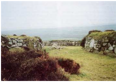
Turf wall cappings at Chysauster (above) and at Tintagel (below), where the florally rich capping offers nature conservation benefits
