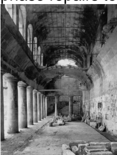
The Gymnasium, Prior Park, Bath; a grant of £275,000
