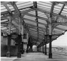
Stately station canopies: Hellifield Station, North Yorkshire; £120,000 for repairs
