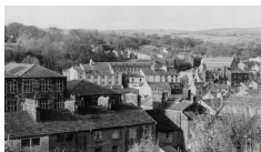
Bacup, Lancs: the focus of a partnership scheme that follows on from a Civic Trust study on the regeneration of the town
