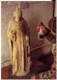
Application of the lime watering treatment to consolidate the surfaces of decaying limestones
