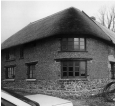
Figure 13 New cob construction in Devon
