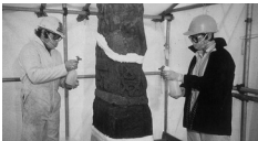
Figure 2 Brethane consolidation treatment
