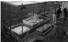
Figure 7 Slaking lime on site
