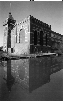
Regent Mill, Oldham: an example of the early 20th-century mill building boom in Greater Manchester, hitherto hardly represented in the statutory list
