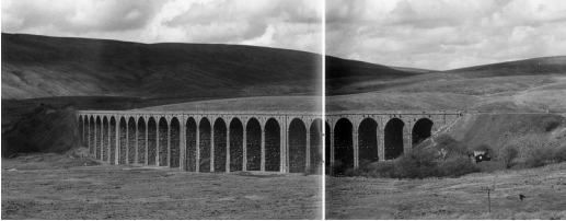
John Crossley's Ribblehead Viaduct, 1875, listed Grade II*, has been restored by the Railway Heritage Trust
