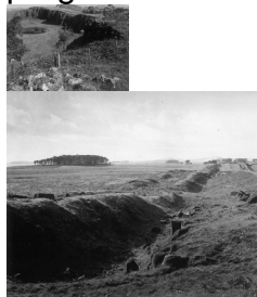
Walltown Crags and Turret, top, and a section of the Vallum, above. The varied landscapes and land uses along the length of the Wall reflect the numerous issues,
