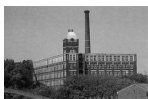
Kearsley Mill, Bolton: a near-complete example of an early 20th-century spinning mill specifically designed for electrically generated steam turbines.
