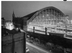
General view of g St Pancras–Kings Cross stations
