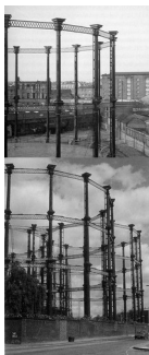
Grade I listed gasholders at St Pancras–Kings Cross stations.
