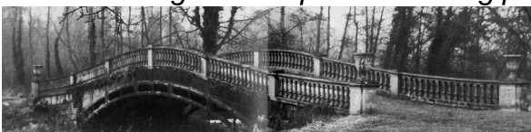
Culford School Bridge, top.
