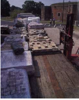
The 40-foot articulated lorry being loaded with materials and equipment en route to West Dean
