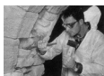
A student chopping out hard cement from one of the ruinettes at Fort Brockhurst Training Centre
