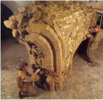
Colin Burns and David Sleight pointing one of the ruinettes at Fort Brockhurst.
