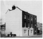
143 Lower Clapton Rd after repairs were completed
