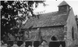
The state of the nave roof before repairs began
