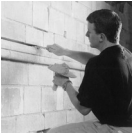
Practical exercise in lime pointing on the ruinette, West Dean College
