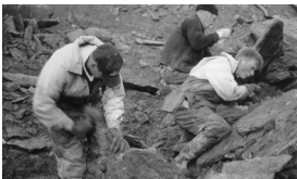
Splitting stone in the quarry – still mainly done by hand
