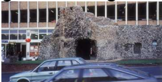
Norwich city walls, trapped between the late twentieth-century ring road and a multistorey car park
