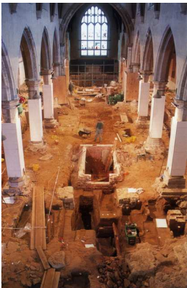
St Nicholas, Sevenoaks: Exhumation of human remains during major interior excavation for new rooms beneath ground level
