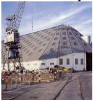
Chatham Naval Dockyard: Covered slips
