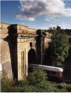
Eastern Portal of Middle Hill Tunnel, Box (1998). 1 K Brunel's engineering feats of the late 1830s still dwarf modern trains
