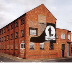
A typical three-storey factory, built in 1891 in Bozeat, Northamptonshire, one of several centres of shoe-making in England which supplied markets in England and the former British Empire
