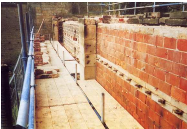
Repair works in progress
