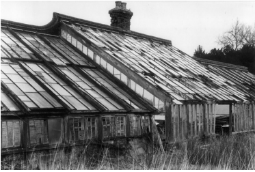
The 1820s Vinery range in 1987, with central display house flanked by vineries. It was repaired in 1993–5, with over 60% of the original timber preserved
