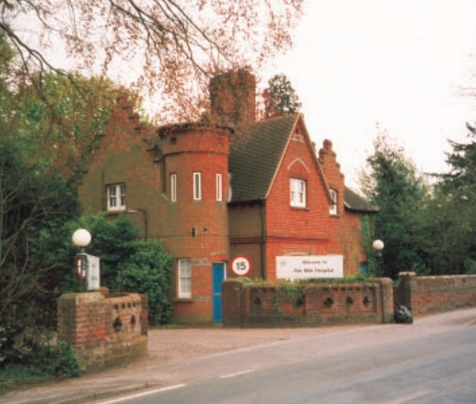
Fairmile Hospital, Wallingford, Oxon (Grade II), the lodge. This former pauper lunatic asylum was built 1868–70. Robert Marnock designed parts of the grounds, which overlook the River Thames and were laid out for the therapeutic use of patients
