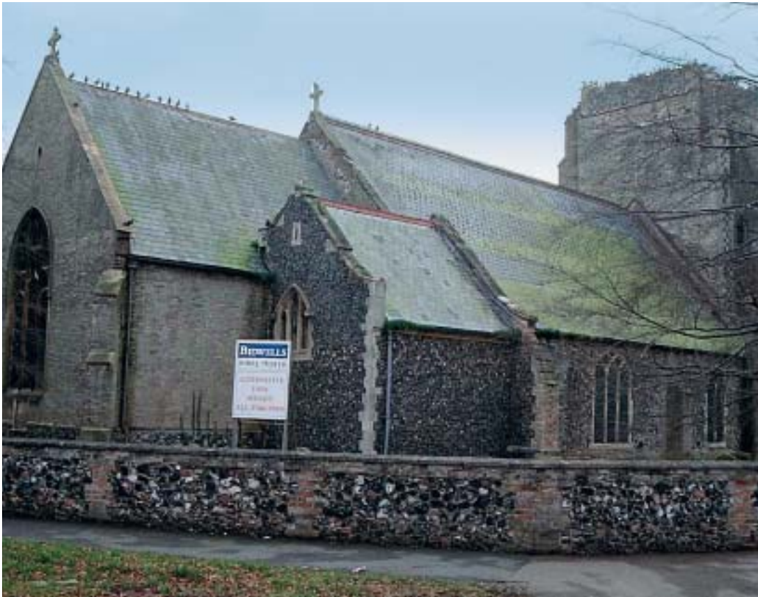
Redundant 14th-century Church of St Mary the Less, Thetford, Norfolk, looking for a new owner
