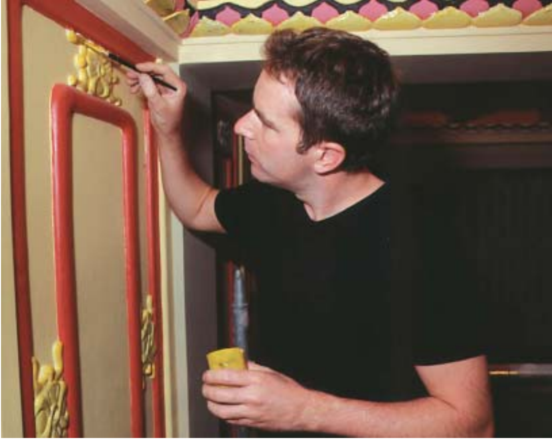
Redecoration of the auditorium ceiling in progress
