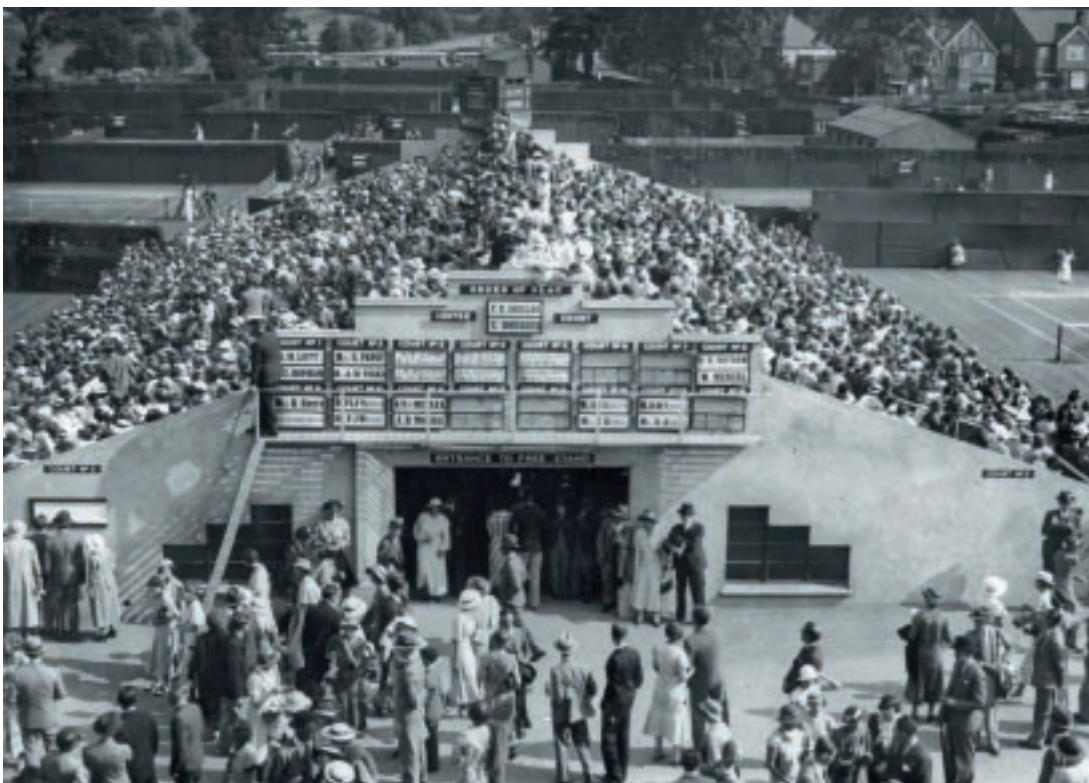
This view from the John Mason Collection, photographed on 30 June 1934, shows the back-to-back stands at the original site of the All England Lawn Tennis and Croquet Club, Wimbledon, Greater London. The stand was constructed using wood re-used from the stands at the original site of the All England Club in Walpole Road, Wimbledon. In 1922, the club was moved to its present location after efforts to extend the former ground failed
