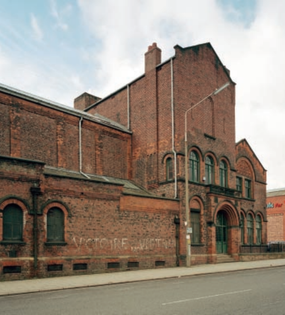
The Manchester Tennis and Racquets Club, designed by George T Redmayne. The building is outstanding as a little-altered example of a rare building type that remains in use for its original purpose
