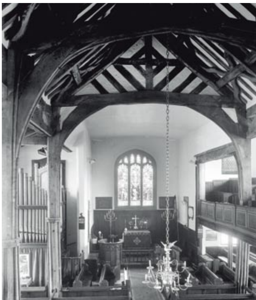
Before and after the uncovering of the arch-brace and timber roof at St Luke's Church, Holmes Chapel, Cheshire (Grade I), recorded by Gerald Sanville during restorations in 1934.
