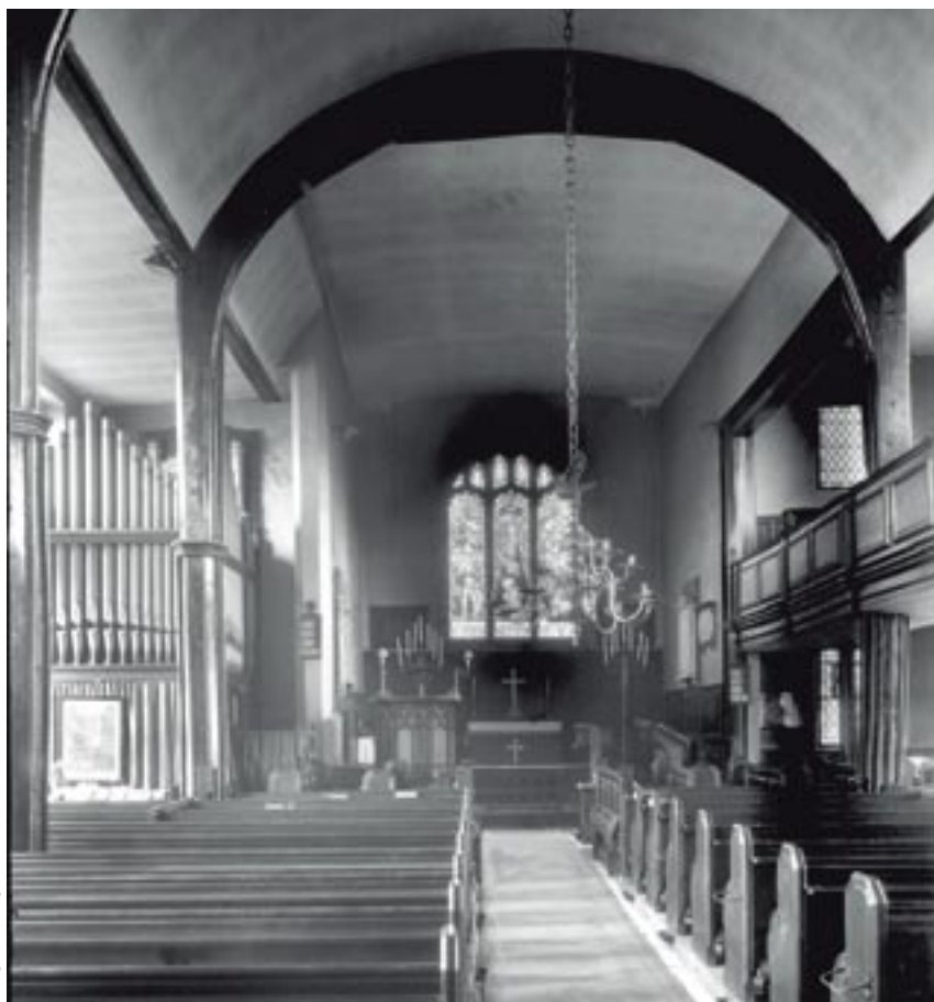
Before and after the uncovering of the arch-brace and timber roof at St Luke's Church, Holmes Chapel, Cheshire (Grade I), recorded by Gerald Sanville during restorations in 1934.
