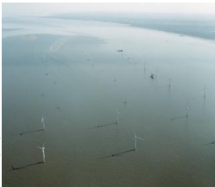
NMR 23501/15 © English Heritage. NMR / Damian Grady
