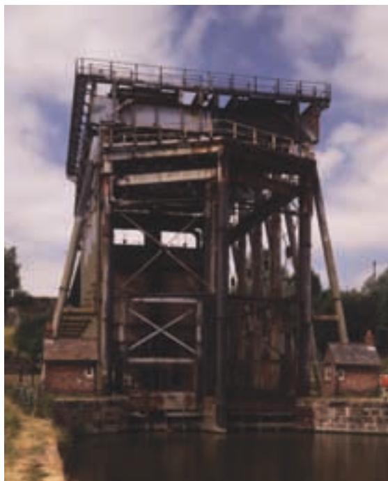
The 1875 Anderton Boat Lift at Northwich, Cheshire, whose £7m restoration to working order was supported with a £3.3m grant from HLF and much careful advice from EH about its conservation.
