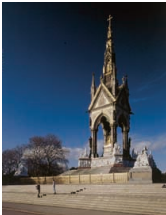
The Albert Memorial repaired and conserved.
