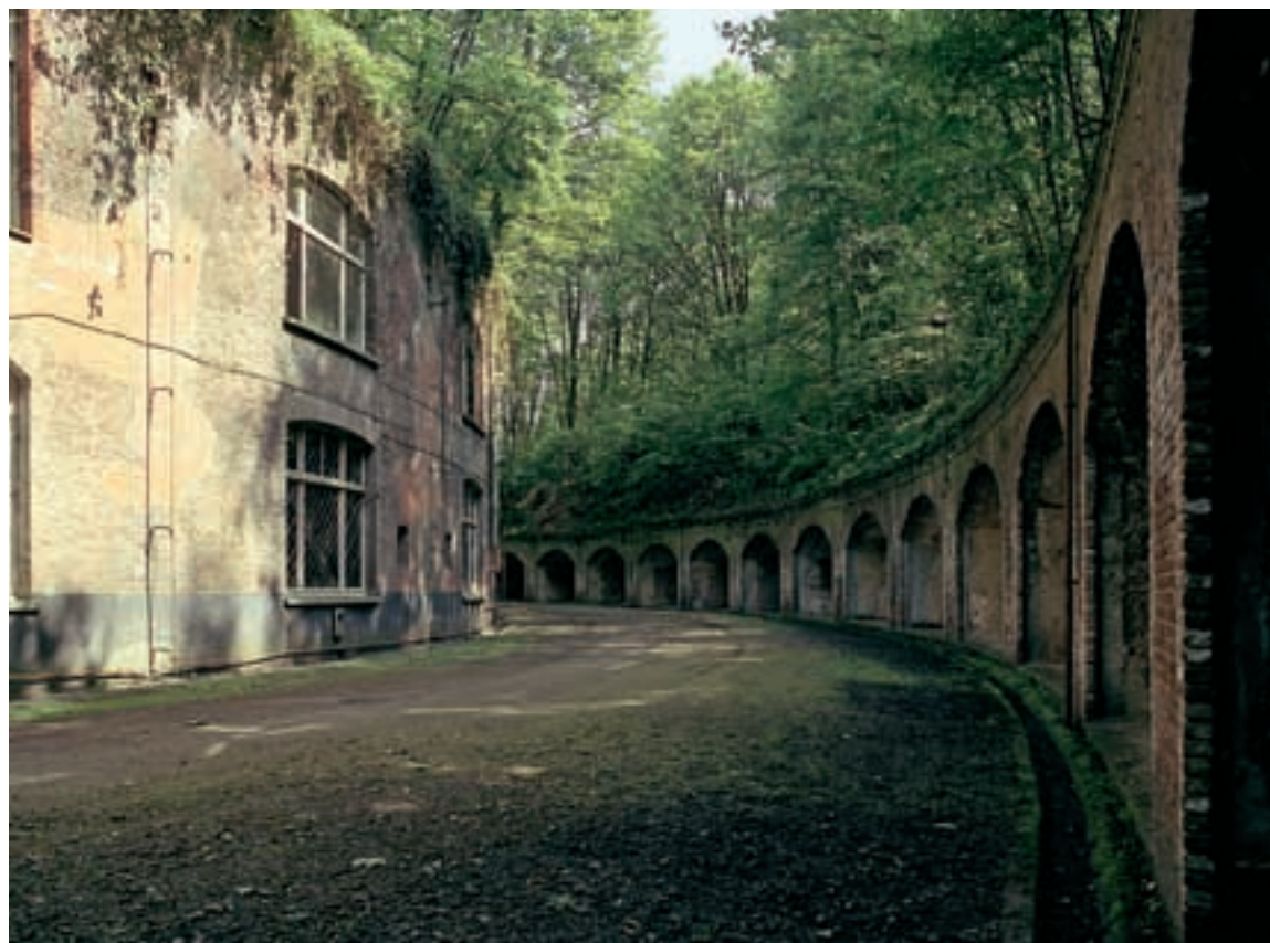
Interior of Fort 4, Mortsel, Belgium, built between 1860 and 1865, as one of a line of forts defending Antwerp. The Crossing the Lines Project has restored and replaced damaged brickwork.
