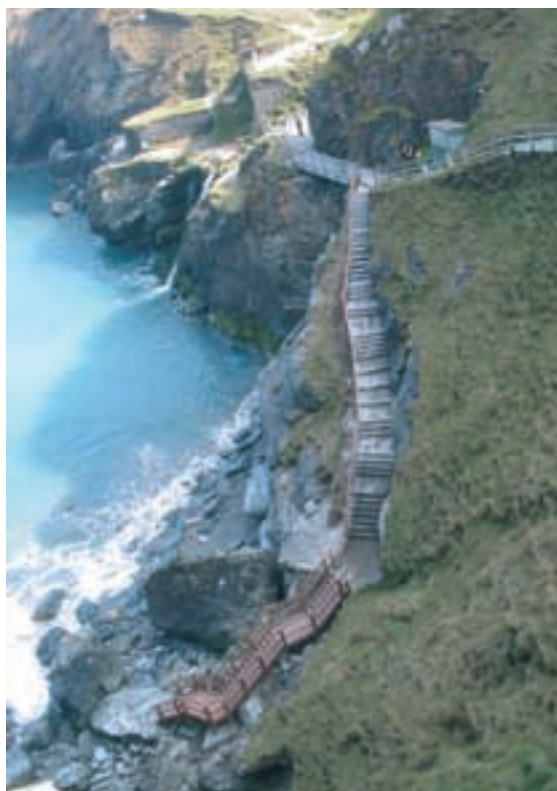
Tintagel Castle, Cornwall: view of the new beach steps installed in 2003 to improve visitor access. The work was carried out as part of a wider Tintagel Regeneration Project part-funded by the European Regional Development Fund (Objective 1) and in partnership with Cornwall County Council.
