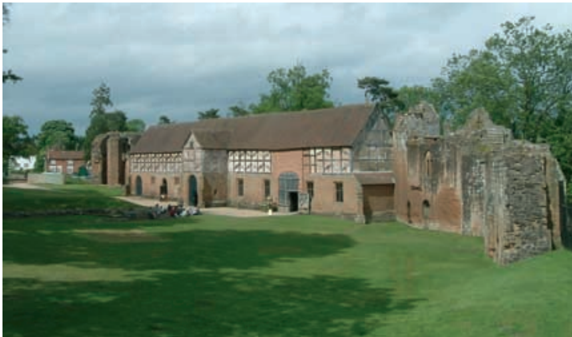
Kenilworth Castle. The 16th-century stables which are part of the scheduled monument.
