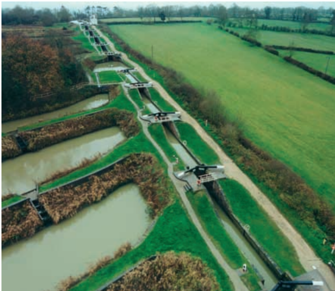
Foxton Locks, Leicestershire. British Waterways and English Heritage have developed a pilot scheme for the streamlined management of this multi-designated historic canal site. As well as being a conservation area, the site contains listed buildings that are still operational, a unique inclined plane classified as a scheduled monument, and associated archaeology, some of it from pre-canal eras.
