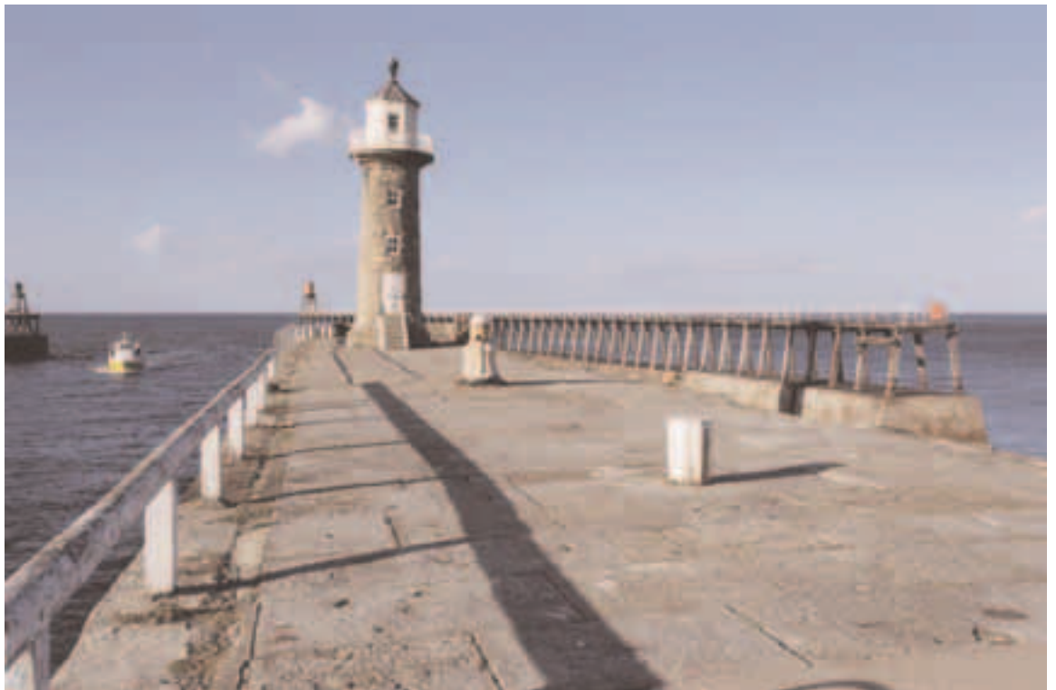
This photograph by Mark Sunderland of East Pier Lighthouse, Whitby, was the winning entry in the Images of England volunteers' competition.
