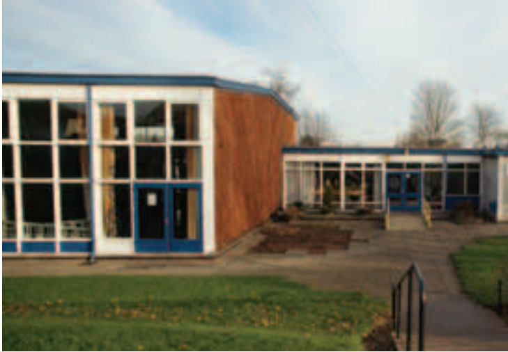
Intake School, Mansfield, 1956, Nottinghamshire County Council Architect's Department. Called the 'Rock 'n' Roll' school for its ability to ride mining subsidence, this was the first school to be built using the CLASP system and is the only post-war school in the county to be listed.
