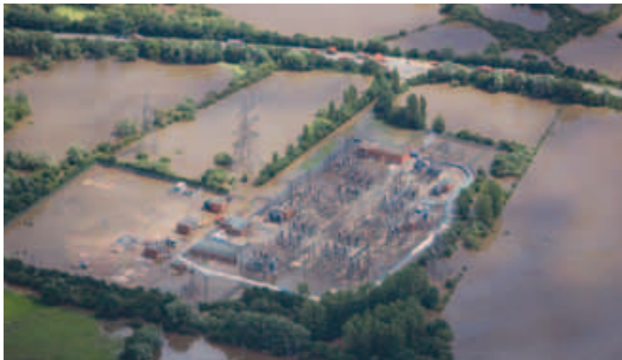
Meeting the infrastructure needs of a brave new world. At the end of July 2007 the emergency services battled to save this vital electricity station on the outskirts of Gloucester from flooding – just one example of the kinds of environmental challenge now facing the over-developed flood plains of southern England.
