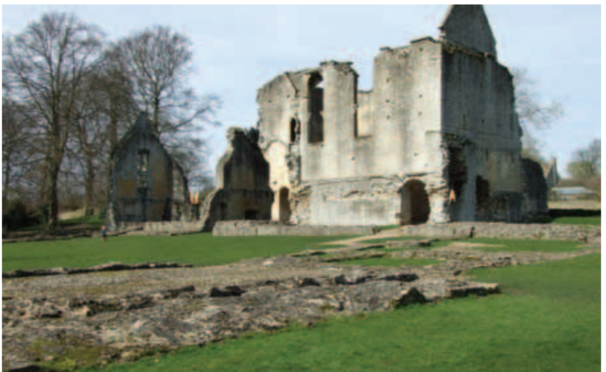
Minster Lovell Hall, Oxfordshire: the traditional way of presenting ruined sites to the public – neatly mown grass, minimal signage and a complete absence of vegetative cover on the masonry.
