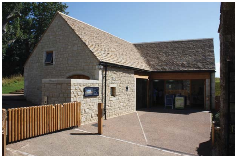
Carisbrooke Castle, Isle of Wight. Although constructed in a modern idiom, the new admissions building clearly owes its form and materials from buildings which preceded it. © Dannatt Johnson Architects
