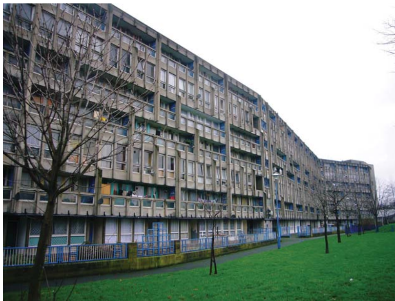
Robin Hood Gardens, Poplar. While not of sufficient architectural or historic interest to merit listing, there is little doubt that this mid-1960s estate could be rehabilitated with handsome results. © English Heritage
