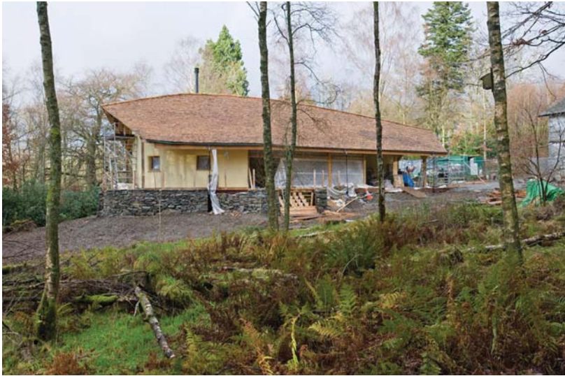
The Footprint building at St Catherine's, Windermere, sits organically in the landscape and has been constructed from straw bales. The project was seen as an opportunity for public involvement from the outset, and numerous volunteers helped with the building. © Sarah Staniforth, National Trust
