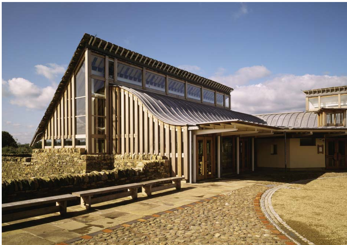
Positioned outside the World Heritage Site and designed in 1992 by Ted Cullinan, the Fountains Abbey visitor centre is large and complex – reception, restaurant, exhibition, shop and meeting/conference room are all housed under one roof and designed with the same architectural character throughout. © NTPL/Matthew Antrobus
