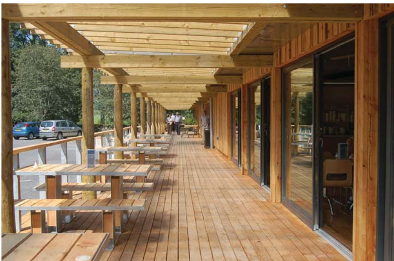
At Sizergh Castle in Cumbria the need to house new visitor facilities away from the medieval castle and buildings led to the commissioning of a low-key modular building. With a lifespan of 30–40 years, it was to be constructed of modern but environmentally sustainable materials and related in character to contemporary agricultural buildings. © Feilden Clegg Bradley Studios.
