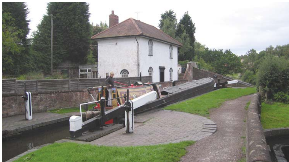
Bumblehole Lock, Wombourne, Staffs. The lock itself is authentic through careful repair and reinstatement; the lock cottage is authentic through minimal investment. © John Yates
