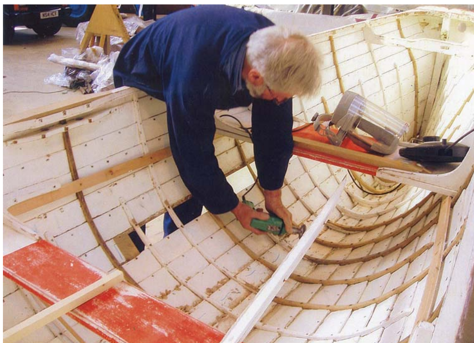
Repairing one of the Newquay Rowing Club's three surviving pilot gigs, the oldest of which dates back to 1812.
