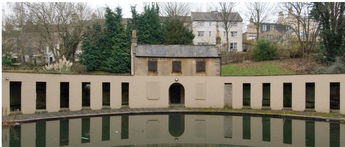
Cleveland Pools, Bath: a rare survival of Georgian outdoor recreational amenity that is now a worthy candidate for restoration to its former glory. © Prince's Regeneration Trust
