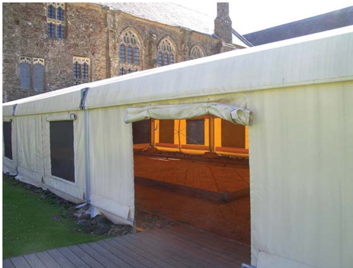
The Frater pavement at Cleeve Abbey protected under a temporary marquee. Its properties of ventilation and insulation were modified during the monitoring period.
