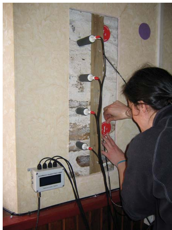
The author applying heat flux sensors to a wall to take an in-situ U-value measurement. © Caroline Rye, ArchiMetrics Ltd
