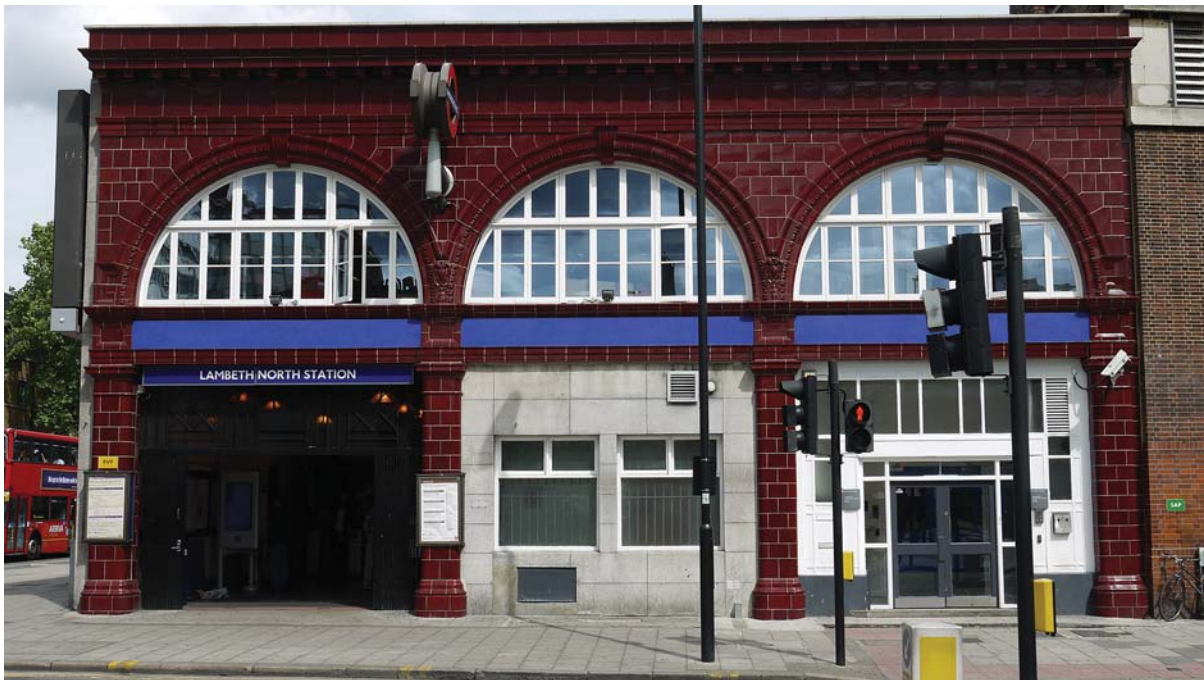
Lambeth North Underground Station (1906), repaired using slip-cast faience. © Alan Baxter & Associates
