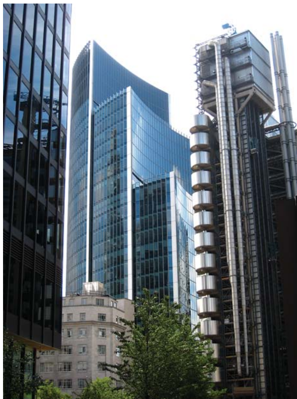
How modern buildings, based on innovative materials and systems, will respond to changing weather patterns is uncertain.
