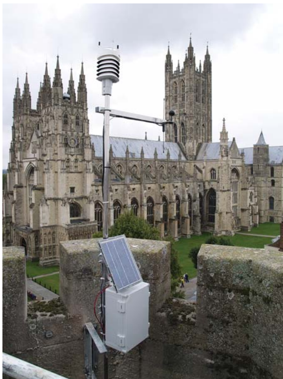
Weather station monitoring the external conditions at Canterbury Cathedral. ©Tobit Curteis
