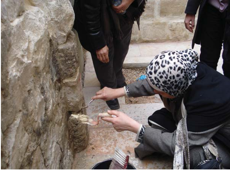
Nablus – pointing training in progress. © David Odgers
