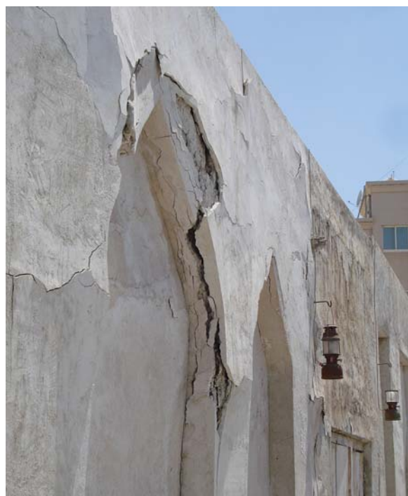
Sharjah – the problems of using cement and gypsum in a dry but humid environment. © David Odgers
