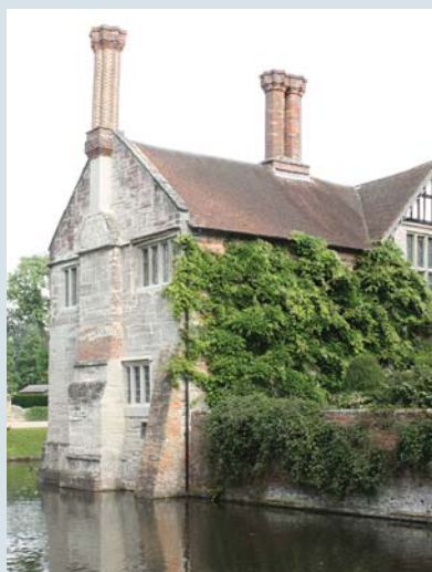
The repaired north-west gable.
