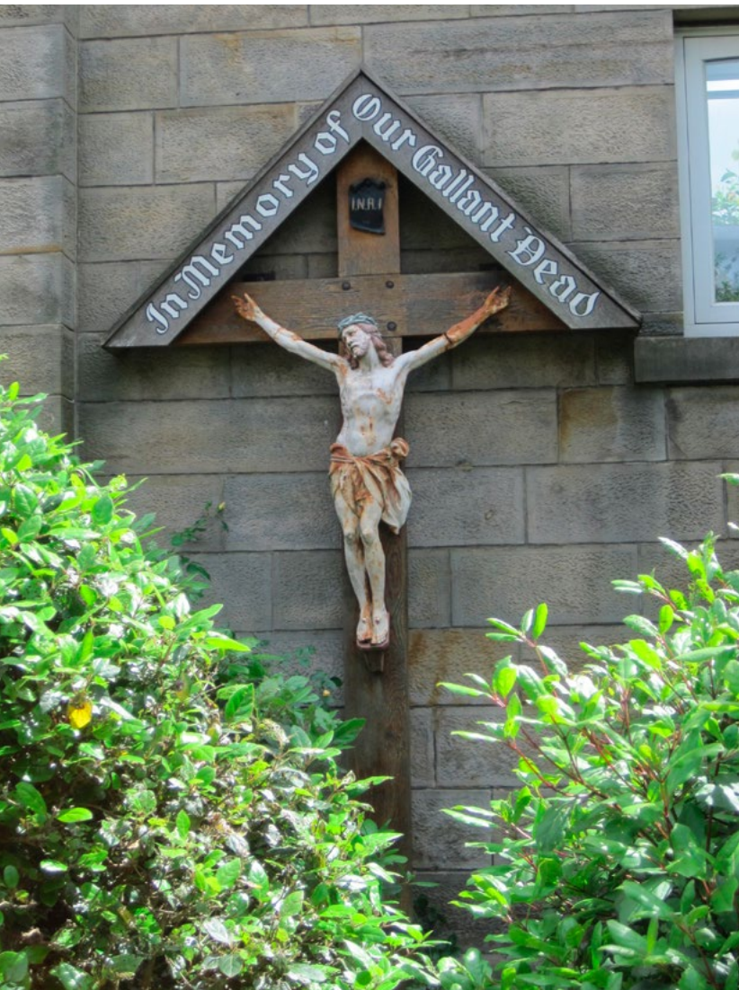
Figure 2.5: St John the Baptist Church, Spalding, Lincolnshire ( WMO/189589 ). A timber inscription panel with raised and incised lettering.
