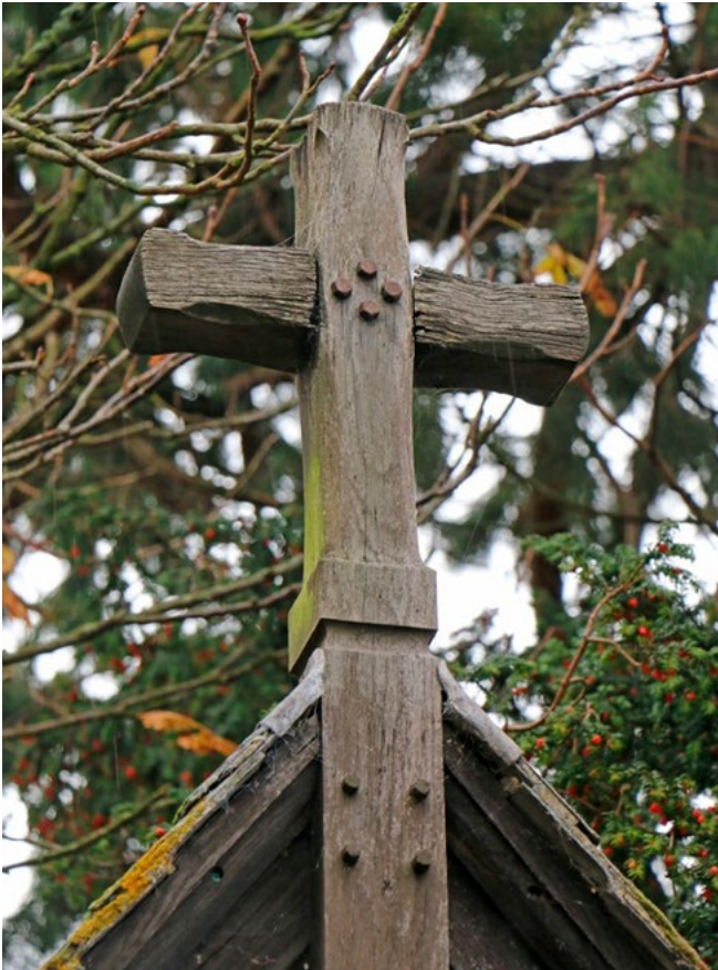
Figure 3.5: This cross is situated at high level at the apex of the lychgate roof. Decay is evident in the cross where the end grain is exposed to moisture at the junctions between the cross bar and the shaft.
