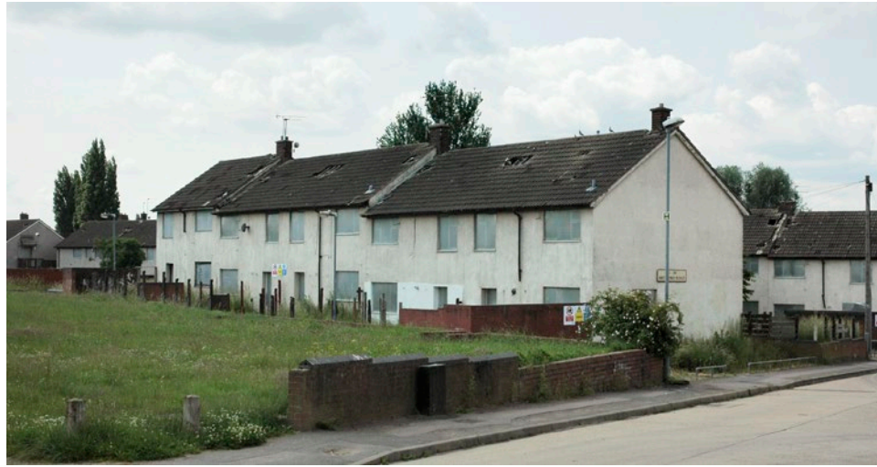
Figure 115 Wimpey 'no fines' houses, Bretford Road, Wood End awaiting demolition in 2013. [© the authors]
