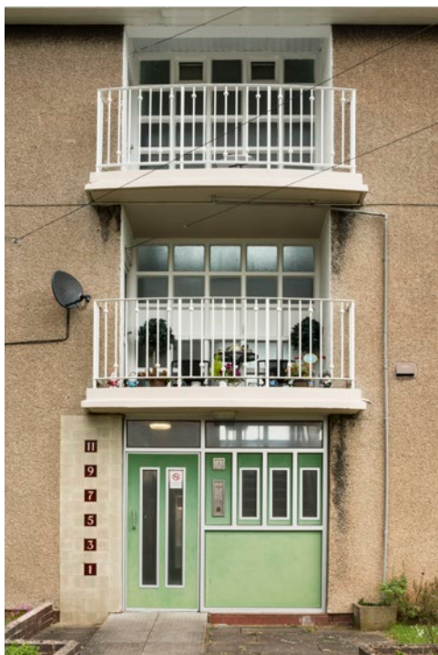
Figure 82 (above) Detail of entrance and balconies to flats, Stonebridge Highway estate (Donald Gibson, city architect and planning officer, 1950–1). A range of coloured tiles, paint colours and balcony balustrades differentiated the entrances. [DP164785]
