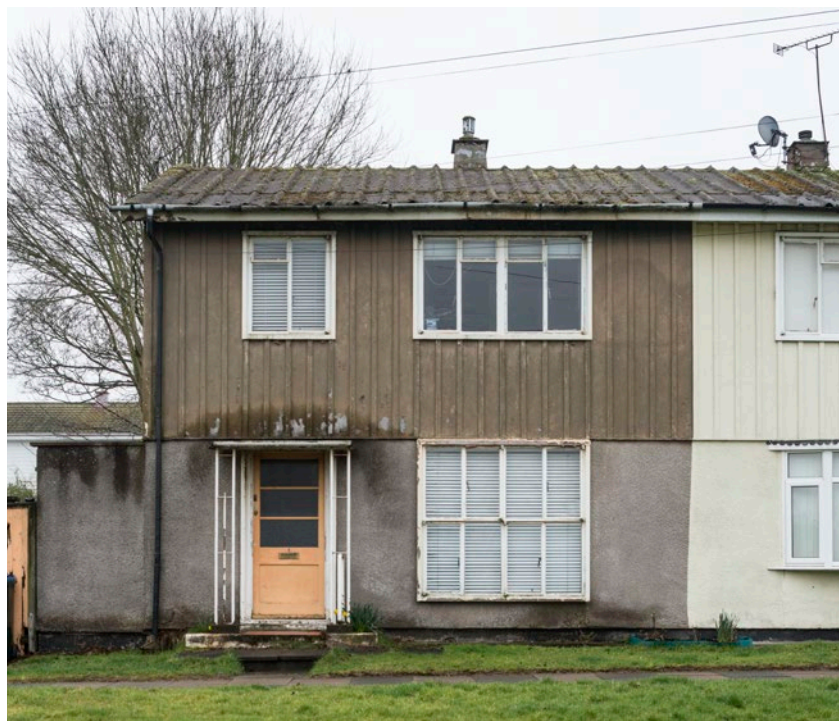
Figure 76 BISF Type 'A' houses, Hancock Green, Canley (Frederick Gibberd, architect, and Donovan Lee, engineer. Layout by Donald Gibson, city architect, 1946–7). [DP172655]
