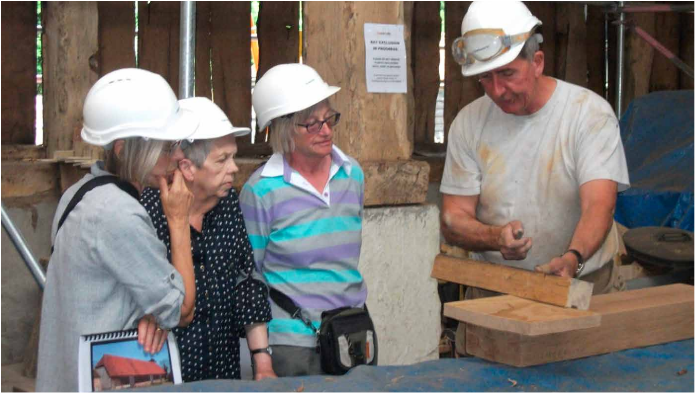
Figure 3 Demonstrating conservation timber repair techniques to visitors.
