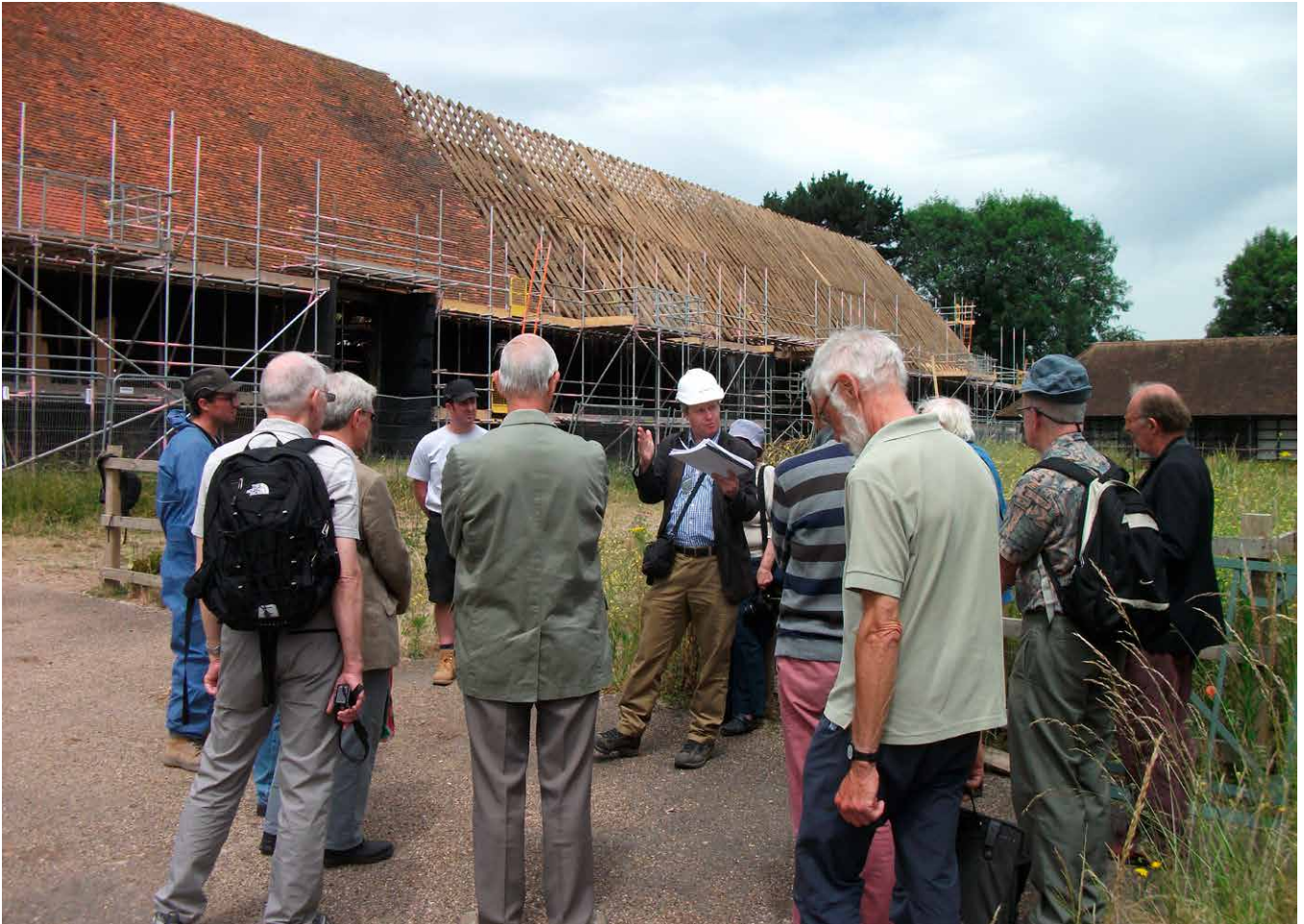
Figure 5 English Heritage Head Curator giving an introduction to members on a hard hat tour.
