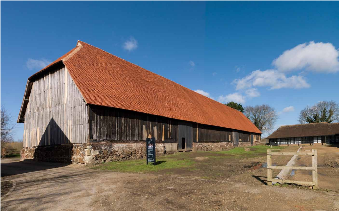
Figure 9 Harmondsworth Barn on completion of the repairs.
