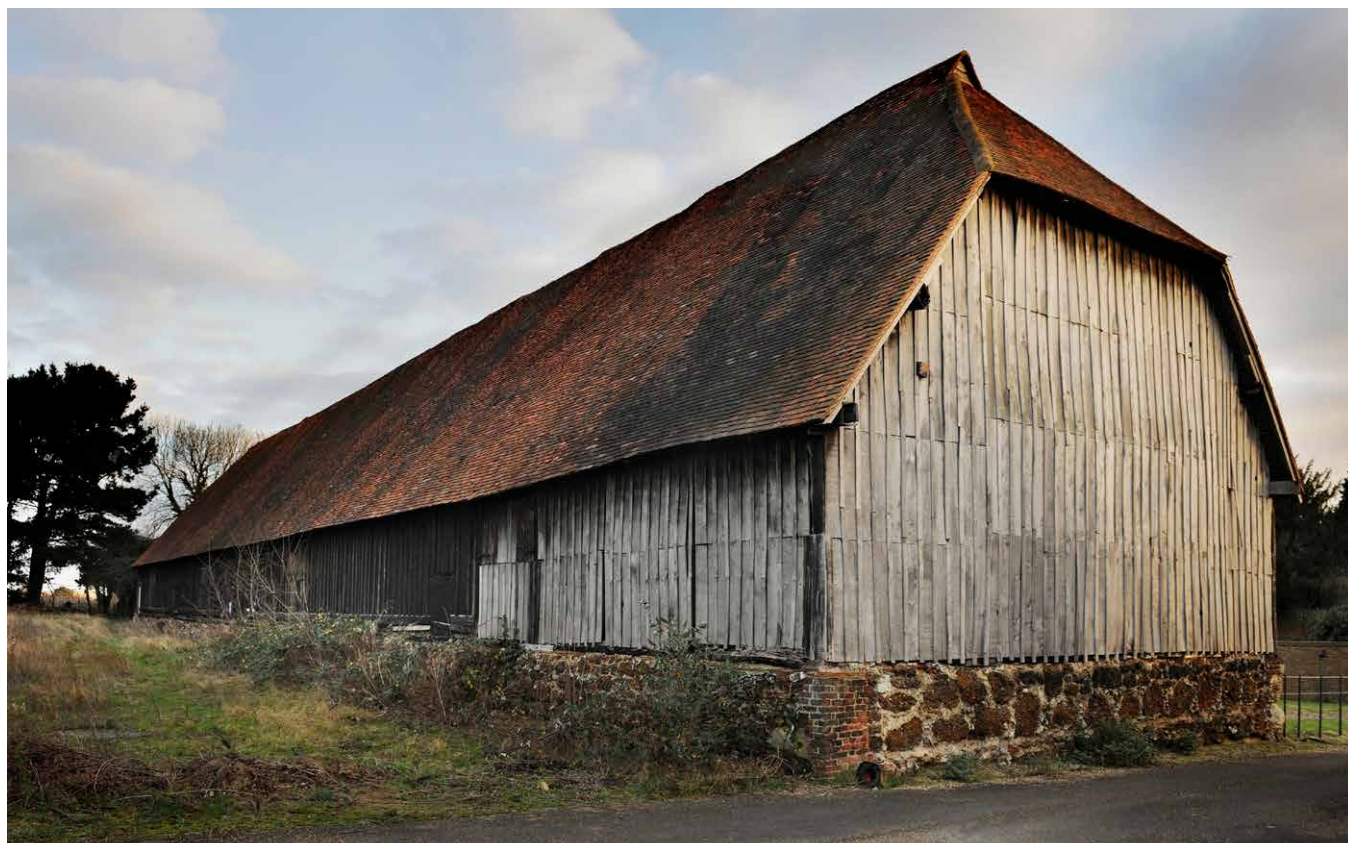
Figure 1 Grade I listed Harmondsworth Barn before the repairs.
