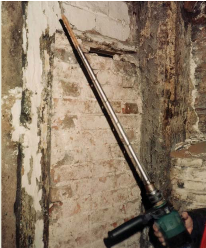
FIG 18 600mm corer used for large timbers; space is needed around the timber before this corer can be used (photo: J Hillam)
