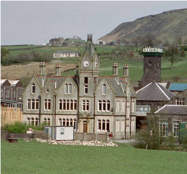
Figure 10 Many otherwise utilitarian factories and industrial buildings were given some architectural panache by the design of their offices and administration buildings, as here at the Dobcross works of Hutchinson and Hollingworth at Saddleworth, Oldham, Greater Manchester, of 1890. Listed Grade II.
