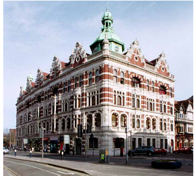
Figure 11 Charter House, Montgomery Way, Portsmouth, Hampshire. Designed as offices for the Pearl Assurance company by C W Bovis in 1891, this grand building is typical of many later nineteenth- and early twentieth-century office blocks which added a note of commercial grandeur to our cities. Listed Grade II.
