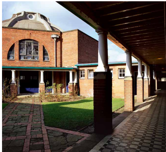
Figure 5 Derbyshire County Council built some of England's most advanced schools. The former Ilkeston Grammar School of 1911-14, by George Widdows, architect to the Education Department and later the county architect, had a large central hall and well-lit classrooms entered from open-air verandahs that (unusually) survive. Thoughtful planning improved both children's education and their health. Listed Grade II*.
