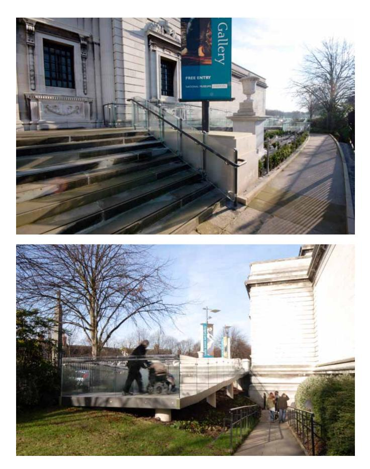
The Lady Lever Art Gallery, Port Sunlight The public entrance was relocated to the west elevation and a new ramp introduced to provide access to the main gallery. A glass balustrade and the use of concrete matching the colour of the limestone cladding limits the visual impact of the new intervention. © Chester Masonry
