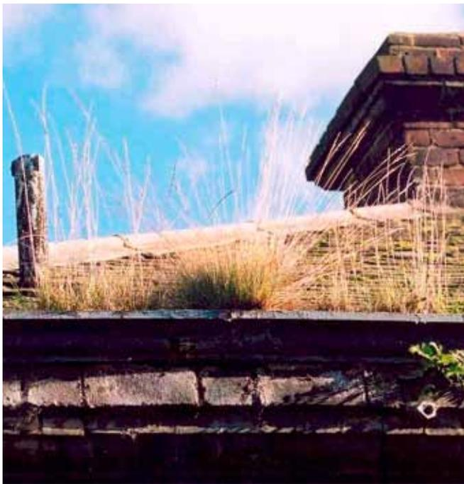
When materials become saturated, frost and the changes in temperature can cause the surface of masonry to wide-laminate and decay. High moisture content in masonry can also result in damage from salts.
