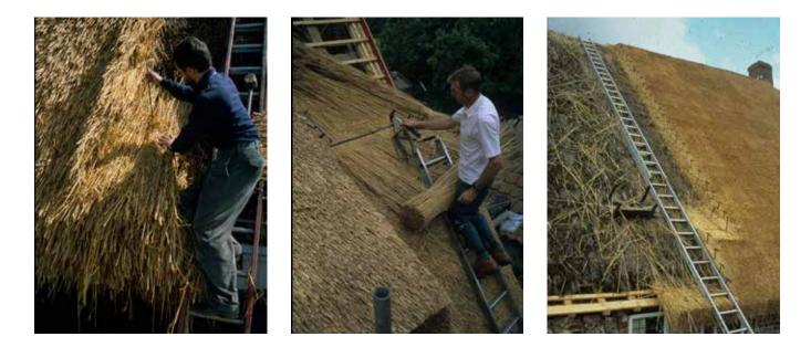
**Figure 2 (left)** Repairs being carried out in long straw.
