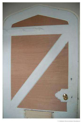
Top left: Draught stripping on a window. Bottom: Insulation was added to this door behind a layer of plywood.
