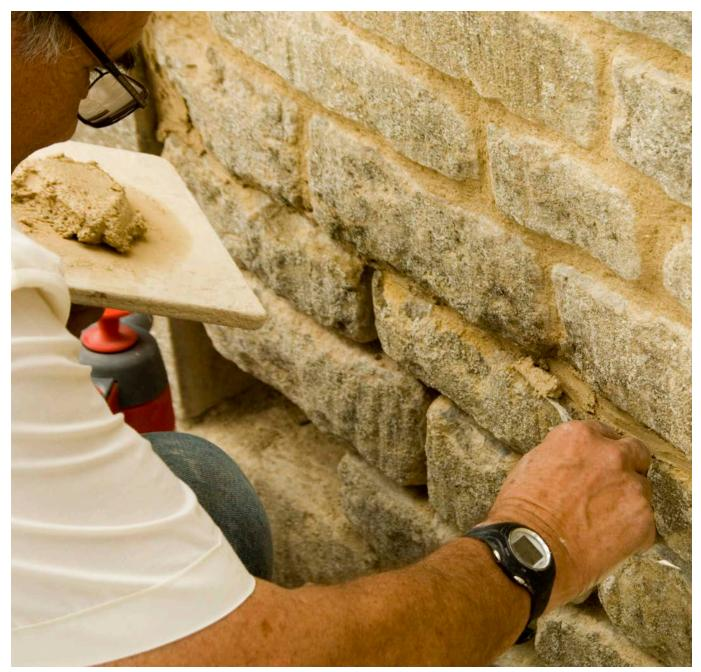
Above: Lime mortar is applied between stones.
