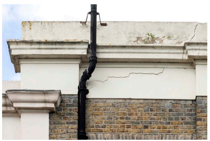
Top: Damage to thatched roof and chimney. Bottom: Cracked masonry render.
