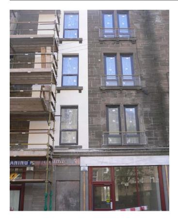
Left: Contrast between part of a building with external wall insulation and part that has none. The visual impact is considerable.
