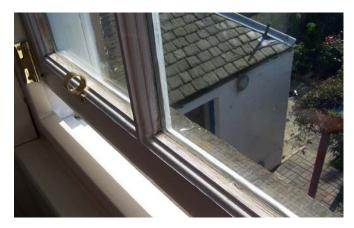
Left: The original timber window frame can accommodate new double-glazing, making the change visually discreet.
