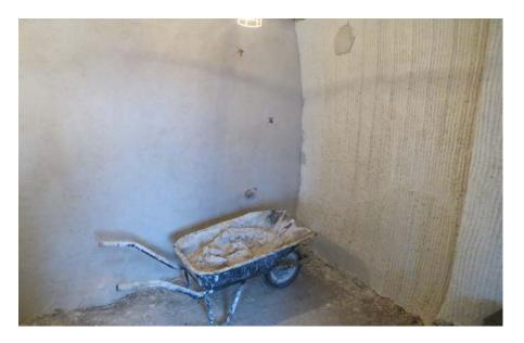
Left: Insulated lime plaster applied directly to a masonry wall.
