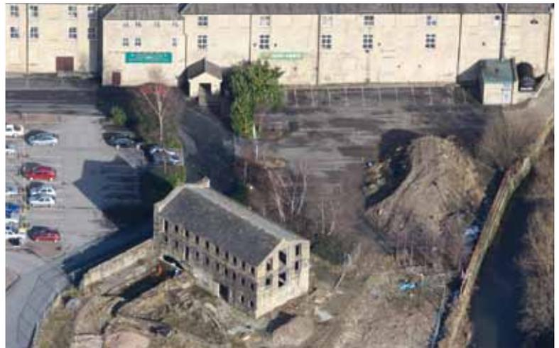
3.31 The construction of Low Mills commenced in 1779 by the Ramsdens of Halifax and was completed in 1780 by Thomas Walsham and William Clayton. The mill was water powered with a dam and goit taken off the River Worth. When the mill came into operation in 1780, it was Keighley's first industrial building and the first cotton mill in Yorkshire.
