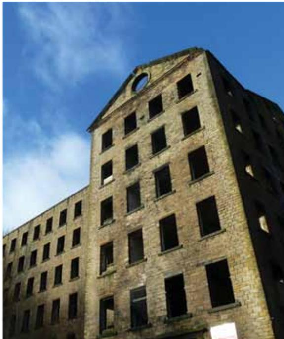
3.45 The mill is of six storeys plus attic and is arranged in an L-Plan. It has 15 x 5 bays with a further 4 bay wing to the right. The mill is the oldest and largest surviving example of a multi-storey, steam powered, iron framed textile mill in the important textile centre of Halifax. Old Lane Mill's attached boiler house and chimney are listed separately from the main mill building. They are also listed Grade II\*.
