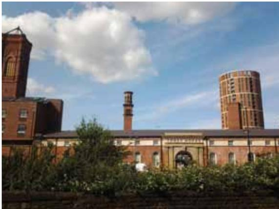
The largest and most ornate tower (constructed in 1899 by Bakewell restored in 1989) is based on Giotto's Campanile in Florence and is known as Giotto Tower. It was used as a dust extraction shaft.
