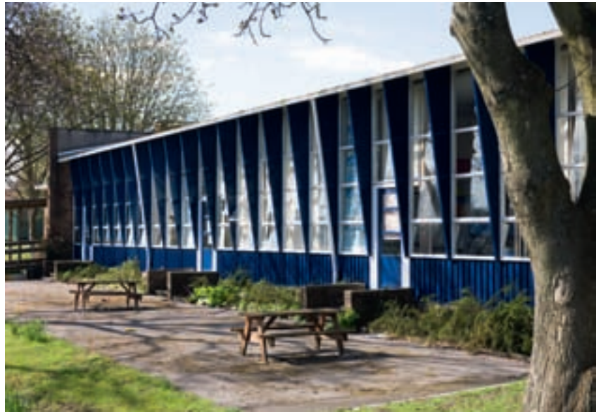
Figure 2 (right) Infant School, Romney Avenue, Lockleaze, Bristol, by Richard Sheppard, Robson and Partners, 1950. This and the neighbouring junior school were the first schools prefabricated of aluminium built as part of a special programme by the Bristol Aeroplane Company, which was looking to diversify after the war. The junior school has been demolished but the infant school survives, much refurbished. [DP057764]
