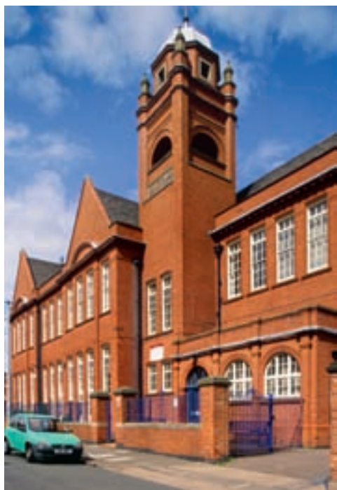
Figure 45 Fosse School, Leicester, of 1898, is one of Edward Burgess's most powerful designs, dominated by its plenum tower. [© Elaine Harwood]
